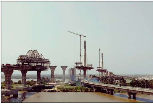
Construction of Pumarejo Bridge in Barranquilla, Colombia
