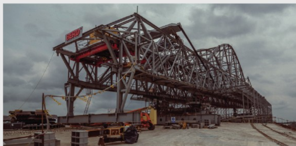
The MSS is being operated by Construgomes
